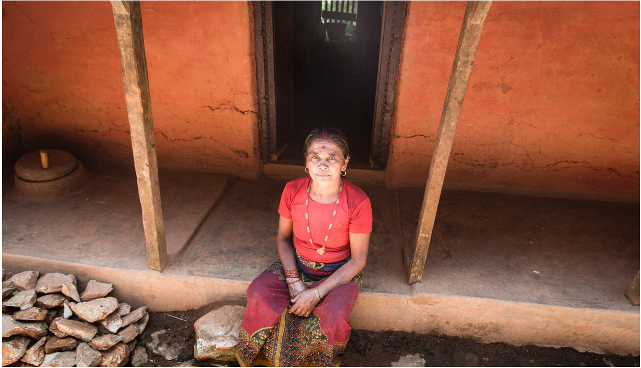
A resident of Makaipur sits in front of her home, which is uninhabitable. Although it looks undamaged, the wall directly behind her has crumbled inward, leaving the roof unsupported. JESSE PESTA/THE WALL STREET JOURNAL
